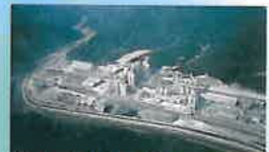
Okke plant of Lafarge Halla cement, Korea
